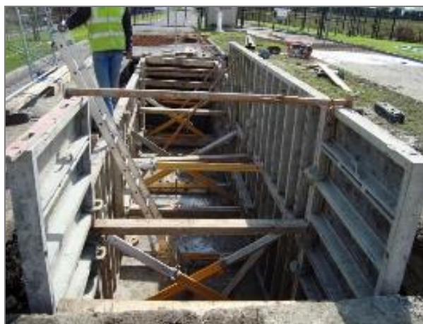
Figure 8.6: Typical Joint Bay under Construction (In Situ)
