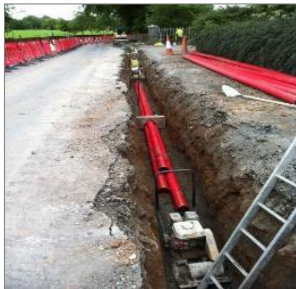
Figure 8.1: Typical 110 kV Underground Duct Installation
