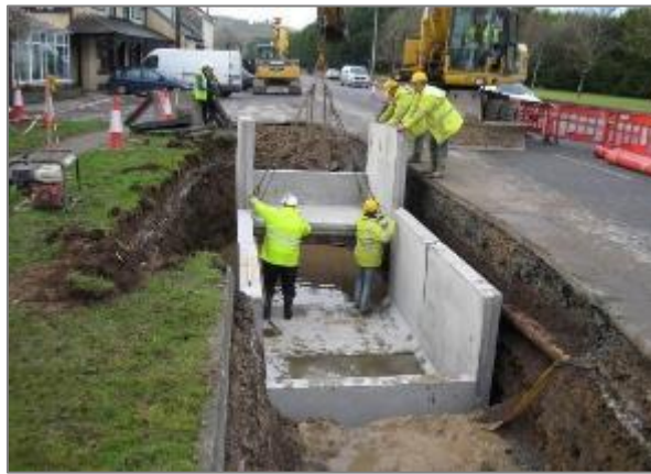
Figure 8.8: Typical Joint Bay under Construction (Pre-Cast)
