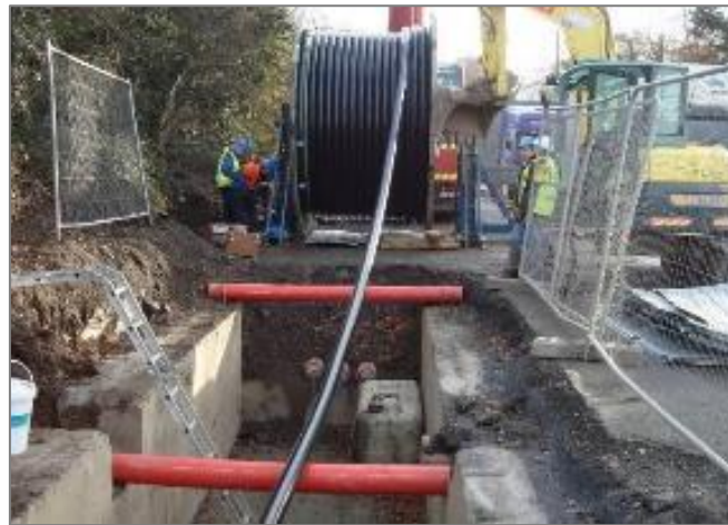
Figure 8.9: HV Cable Pulling Procedure (Typical Drum Setup)
