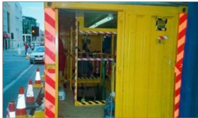
Figure 8.10: HV Cable Jointing Container
